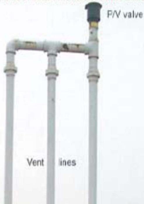
Three vent lines manifolded into one.
